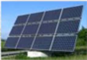
Ground PV Solar Array
